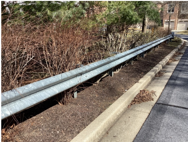
Metal guardrail overview
