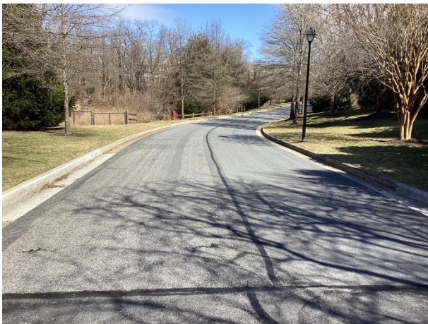
Asphalt pavement street overview
