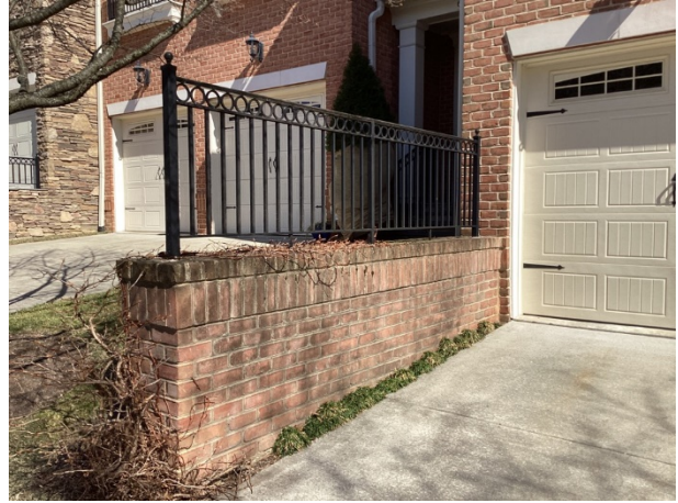
Aluminum railing overview
