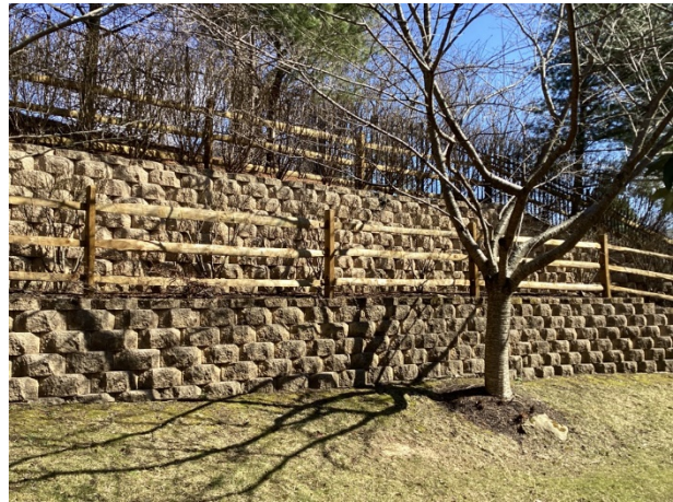
Masonry retaining wall
