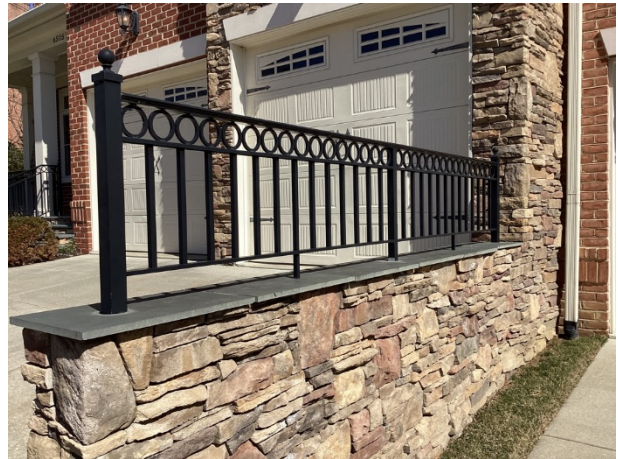
Aluminum railing overview
