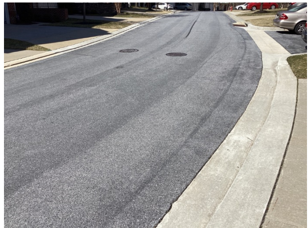
Asphalt pavement street overview - Note minor wear
