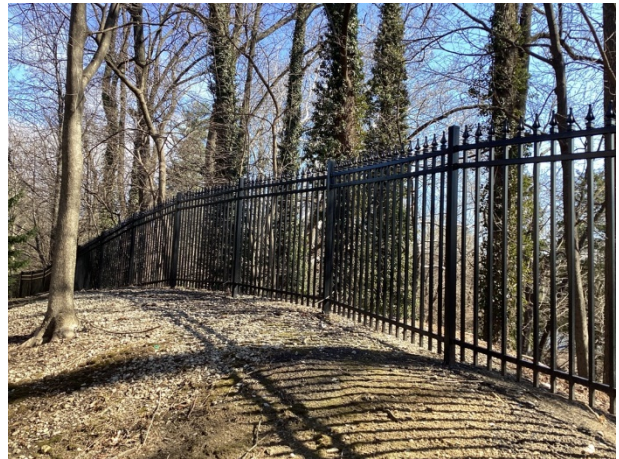
Aluminum fence overview
