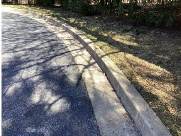
Concrete curb and gutter
