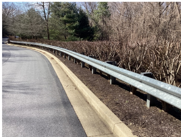
Metal guardrail overview
