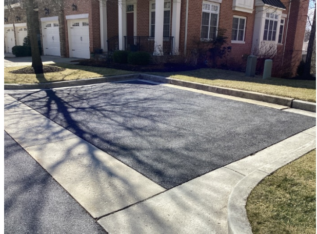
Asphalt pavement parking pad overview
