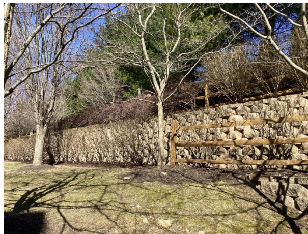
Masonry retaining wall
