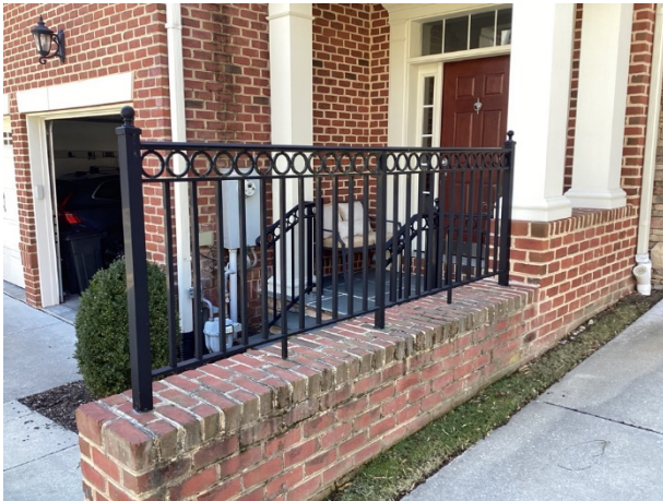
Aluminum railing overview
