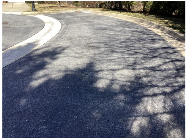
Asphalt pavement parking pad overview
