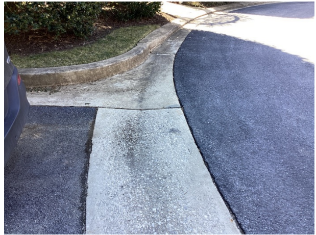
Concrete curb and gutter
