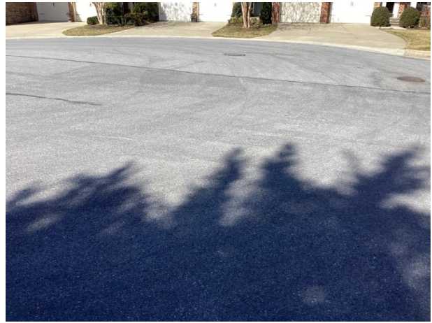
Asphalt pavement street overview
