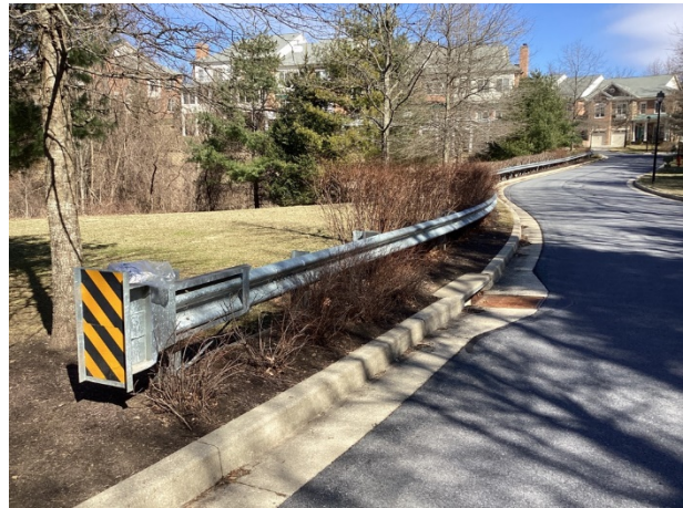
Metal guardrail overview
