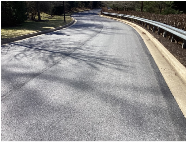
Asphalt pavement street overview
