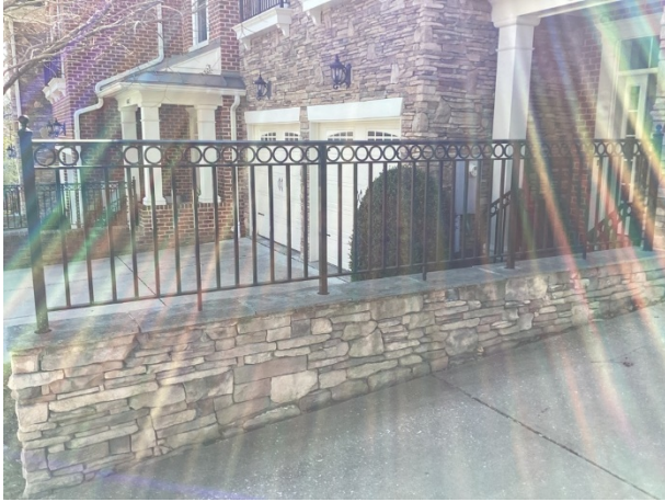
Aluminum railing overview
